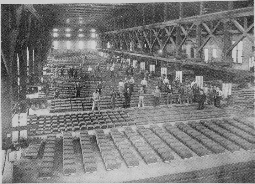
This inside view of the mammoth foundry of the Columbus Iron Works Company is shown in the above photo.
